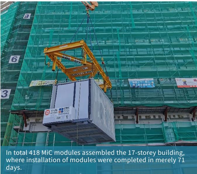
In total 418 MiC modules assembled the 17-storey building, where installation of modules were completed in merely 71 days.
