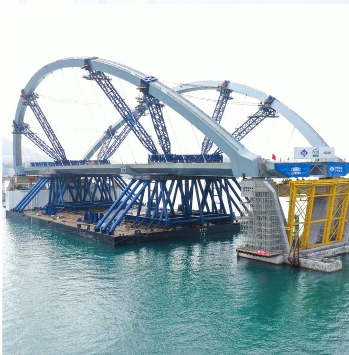
Erection of the steel arch bridge by "Float-over" method
