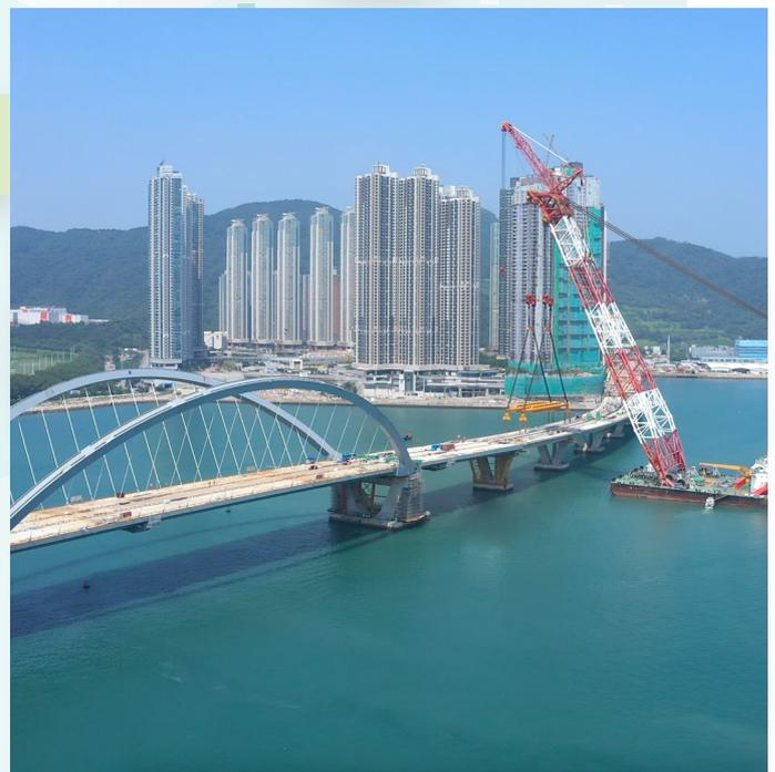
Erection of concrete box girder by full-span lifting method
