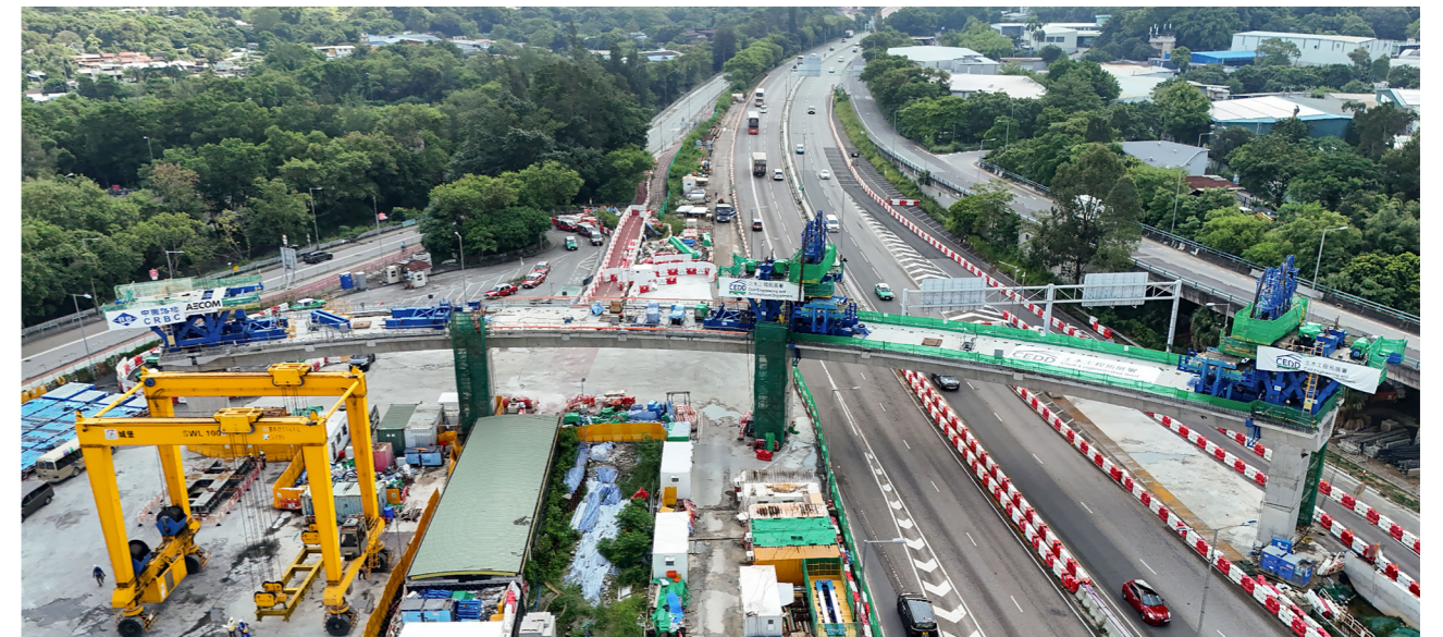
Aerial View of Bridge ST01 constructed by Full-Span Deck Erection Method
