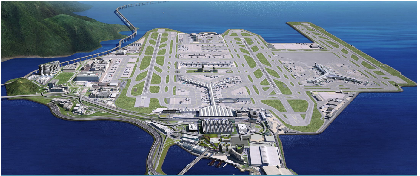
The completion of pavement works on the 3,800-metre-long and 60-metre-wide Third Runway
