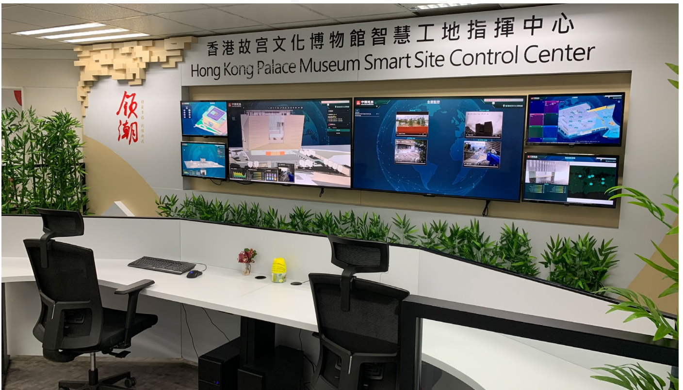
Smart site Command Center
